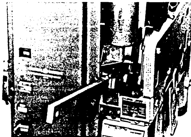
FIG. 11 — MAINTENANCE HANDLE INSTALLED ON CAMSHAFT EXTENSION
