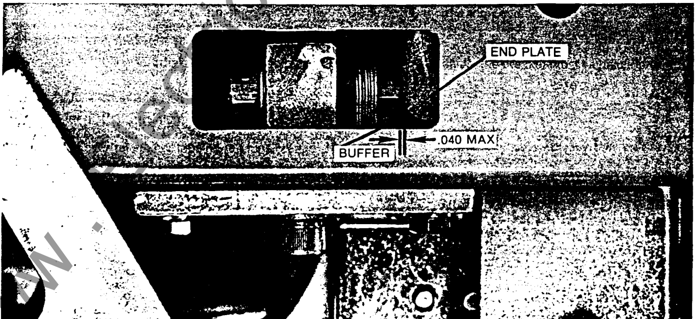
FIG. 41 — BUFFER/END PLATE RELATIONSHIP—BREAKER OPEN
