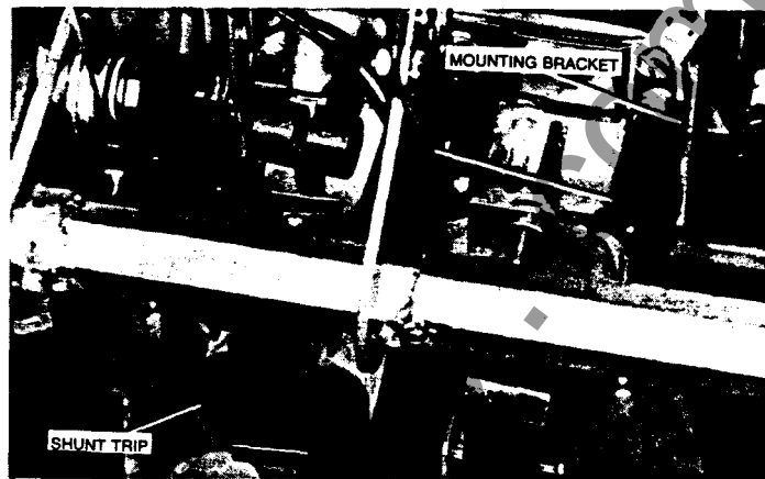
FIG. 29 — SHUNT TRIP AND UNDERVOLTAGE MOUNTING
