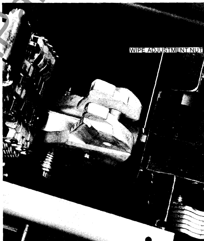
FIG. 47 — 1600 AMP CONTACT STRUCTURE
