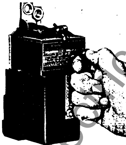
FIG. 102 CHECKING TRAVEL DISTANCE OF SERIES OVERCURRENT TRIPPING DEVICE.
