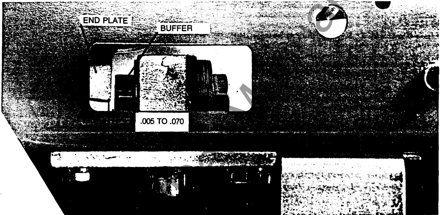
FIG. 40 — BUFFER/END PLATE RELATIONSHIP—BREAKER CLOSED
