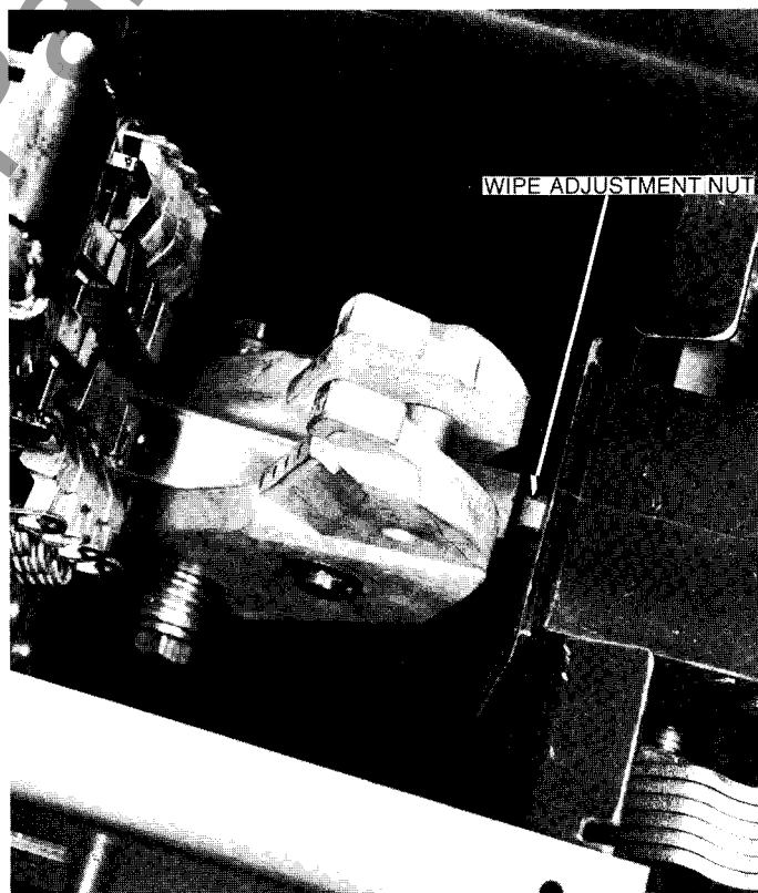
FIG. 47 — 1600 AMP CONTACT STRUCTURE
