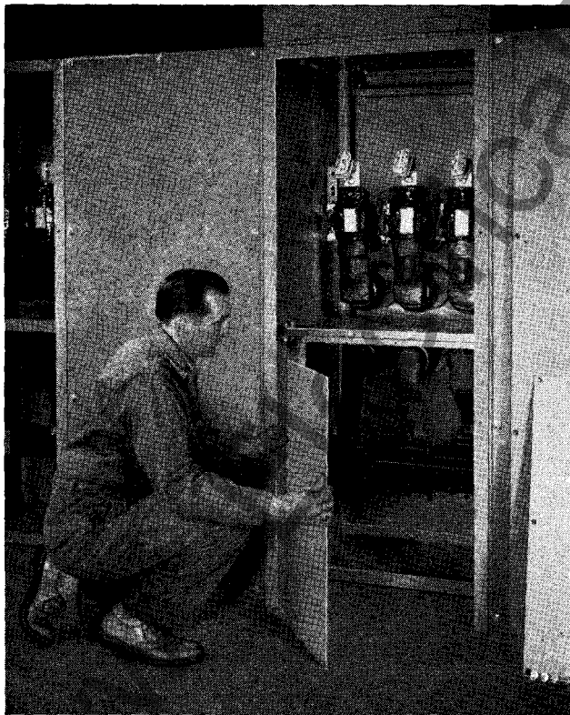
FIG. 37. Removing Barriers of Main Bus Compartment. (Busses are also accessible from breaker side of housing by removing bolted section of barrier).
