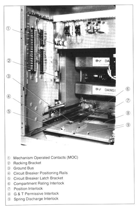
Figure 4: Circuit breaker interlocks
