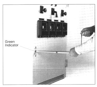
Figure 8: Racking—circuit breaker in test position
