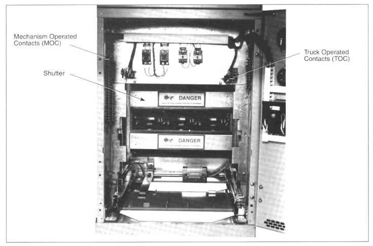
Figure 13: Circuit breaker cell—shutter closed
