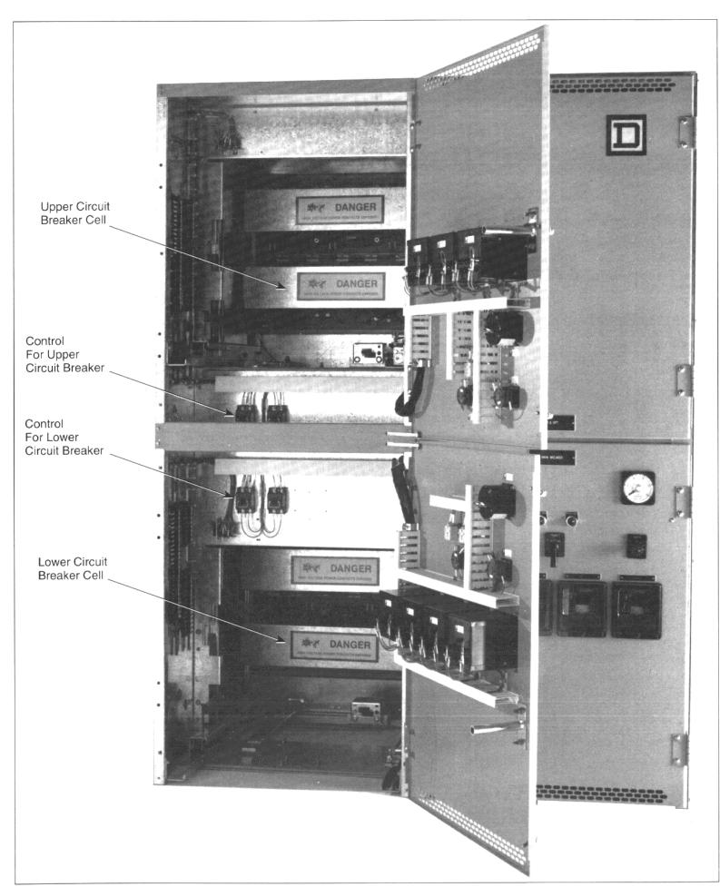
Figure 1: Circuit breaker cells without circuit breakers
