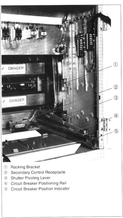
Figure 5: Shutter assembly and interlocks
