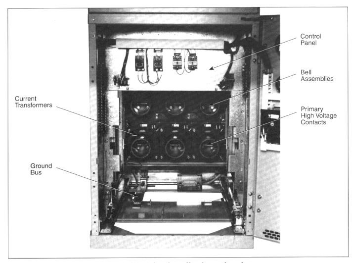
Figure 12: Circuit breaker cell—shutter forced open
