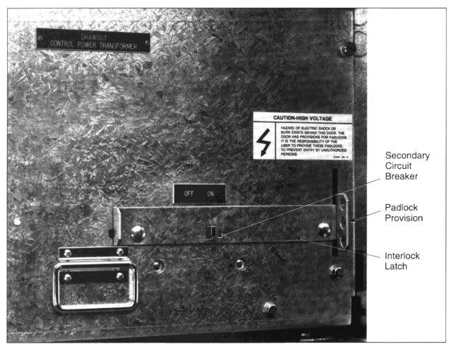
Figure 18: Control power transformer—secondary circuit breaker interlock
