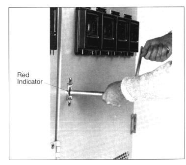
Figure 9: Racking—circuit breaker in connected (operating) position
