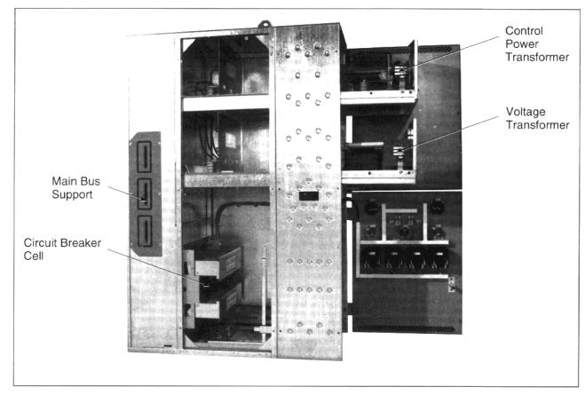
Figure 15: Drawout units in withdrawn position
