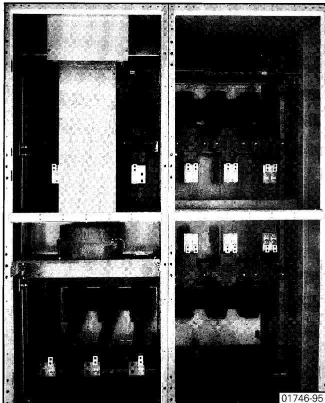
Figure 26. Typical Cable Termination Compartments (Unit on left has top breaker cables exiting top, and bottom breaker cables exiting top through "chimney" or trough. Unit on right has top breaker cables exiting top and bottom breaker cables exiting bottom.)
