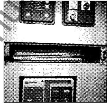
Secondary Control Terminals
