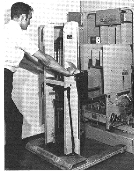
14 Replace contactor, either using jiffy bar or fork lift truck. Push contactor to rear of cell.
