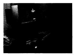
SAMMS-LVE and SAMMS-MVE units are tailored to the needs of across-the-line non-reversing applications. SAMMS-LVX and SAMMS-MVX units are programmable to provide the control logic for all common starter arrangements, including:
