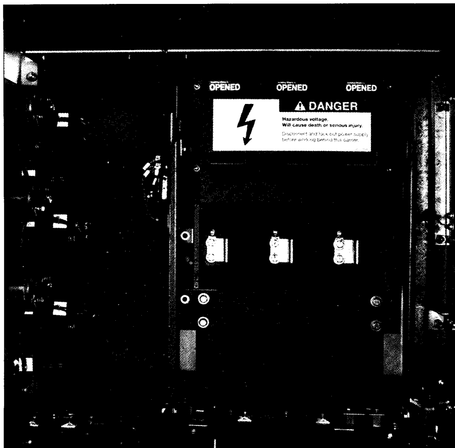
Controller Interior — Insulated Shutters Cover Line Side Stabs when Carriage is Withdrawn
