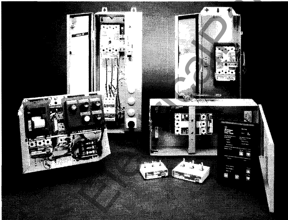
IQ Energy Sentinel Applications Left to Right: MCC Starter, Enclosed Starter, Enclosed Breaker and Busplug
