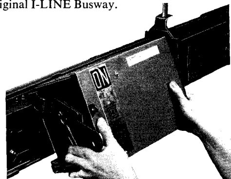
INSTALLING PLUG-IN UNIT
