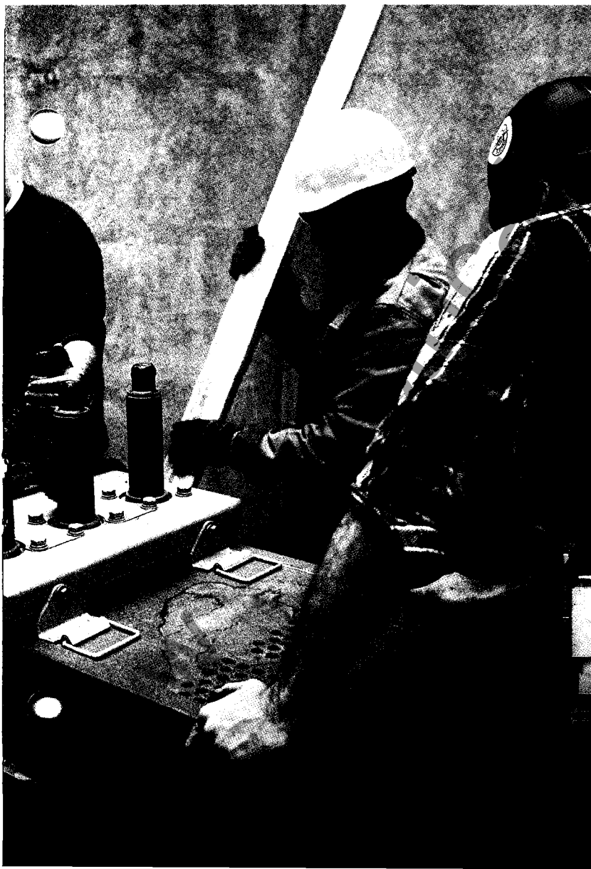
GE MAGNE BLAST™ circuit breaker being replaced with a modern, retrofit model.
