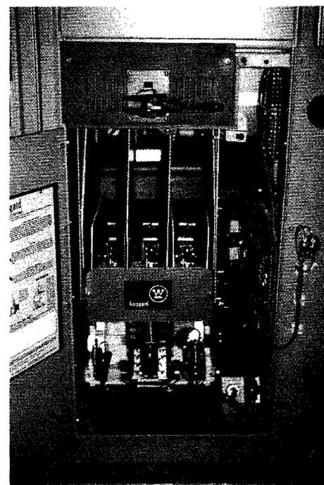
26 in. wide 50L2 air break design, with SJO Vacuum Contactor Retrofit installed. (Power fuses not installed).
