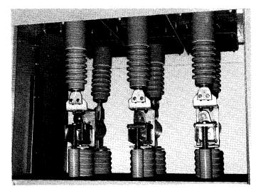
All components at line potential are contained in the high voltage section and are completely isolated from the control compartment. Porcelain entrance bushings are attached to the roof assembly by bolt and compression type clamps. Removal or replacement does not disturb existing breaker adjustments. Bushing current transformers mount on the entrance bushings. The accuracy class required determines the
