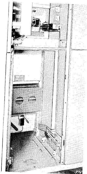
Fig. 23. Indoor and Outdoor: 5 KV Breaker Housing with MOC Sw
