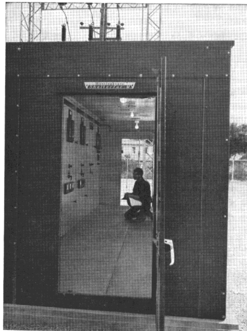
fig. 30: Close-up of sheltered service aisle for personnel and equipment.
