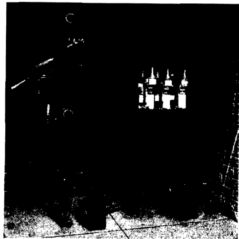
FIG. 3—REMOTE-CONTROL WALL-MOUNTED TYPE F-11 OIL CIRCUIT-BREAKER
