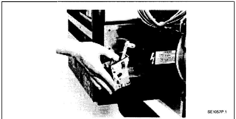
Figure 83 Bypassing the Cell Door Interlock
