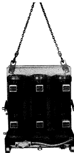
Figure 2: Circuit breaker lifting
