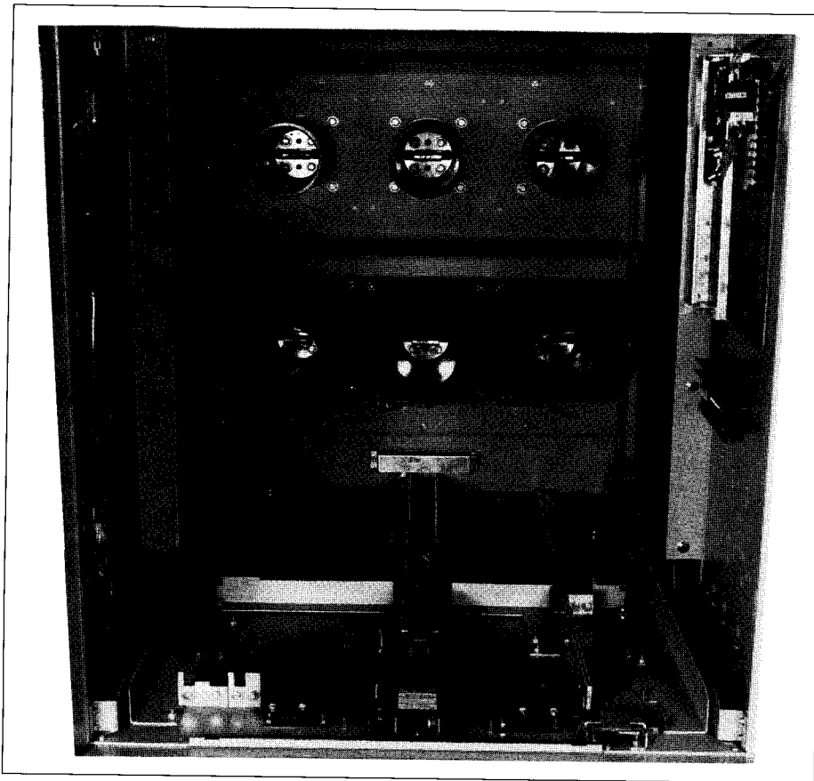
Circuit Breaker Cell Interior (CT Barrier Removed and Shutters Open)
