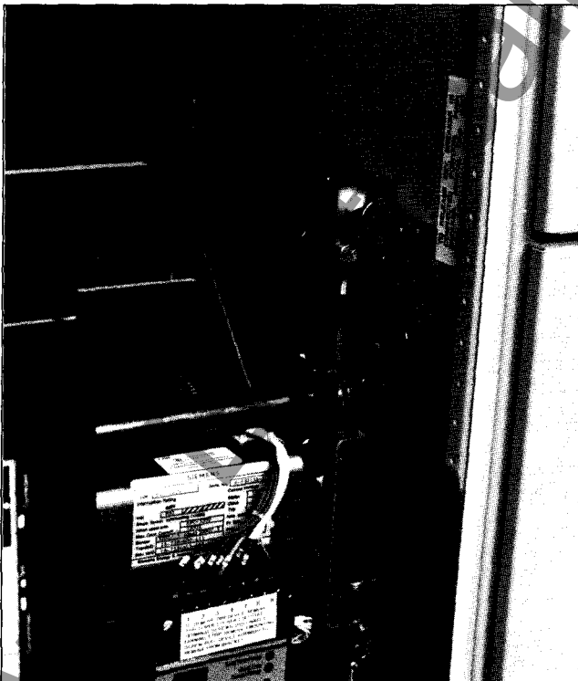
Figure 12. Key Interlock Mounted in Circuit Breaker Compartment
