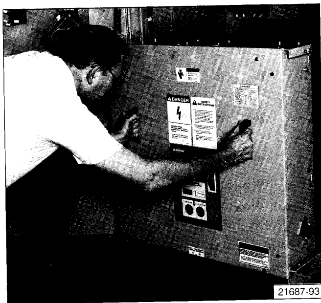
Figure 4: Removal of Circuit Breaker.
