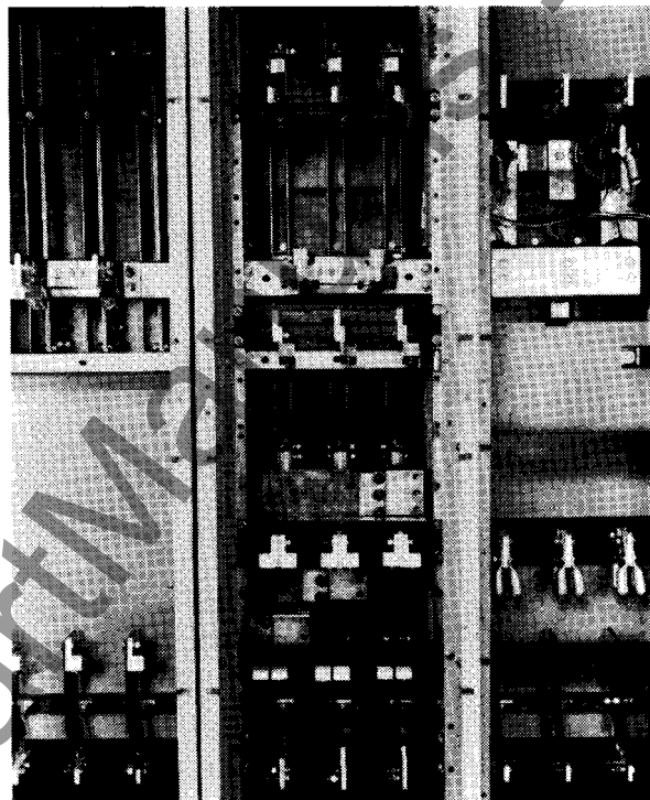
Figure 3. Rear View Showing Bolted Copper Main Bus and Bus-Cable Compartment Barriers.
