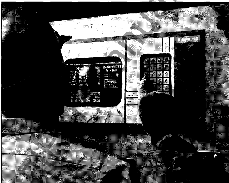
Power Monitor display and monitoring unit with sealed input panel
