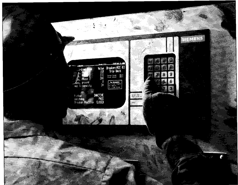
Power Monitor display and monitoring unit with sealed input panel
