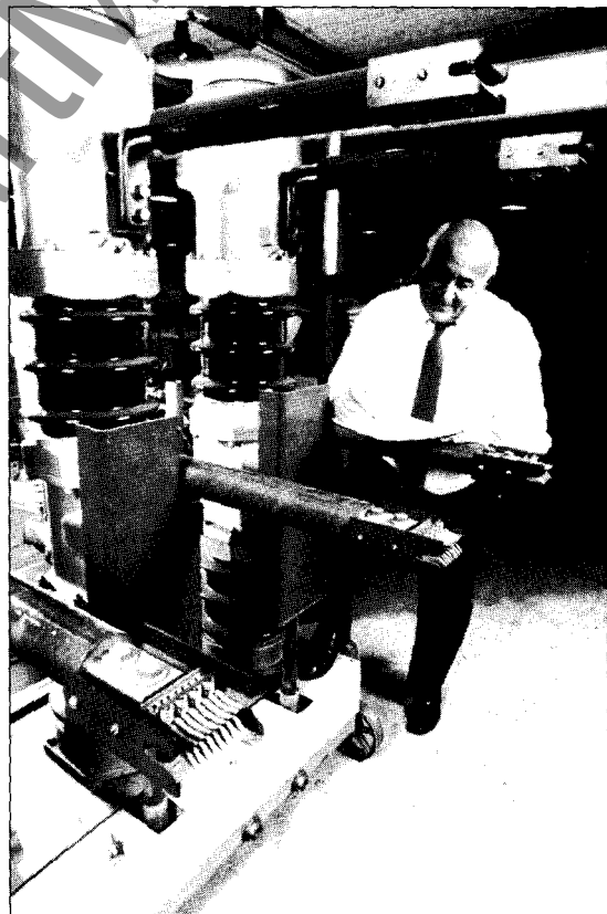
Technician inspects a 1,200 A minimum oil breaker unit being readied for retrofit. The original trucks of the units are stripped of springs, motors and gears, leaving only the bayonette-type connectors.
