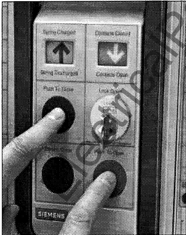
Discharging energy from the stored energy mechanism without closing contacts.
