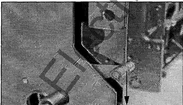
2. Pull the release lever down to the release-disengaged position. (Illustrated beneath padlock device.) If the breaker contacts are closed, pulling the release lever down will trip the breaker.
