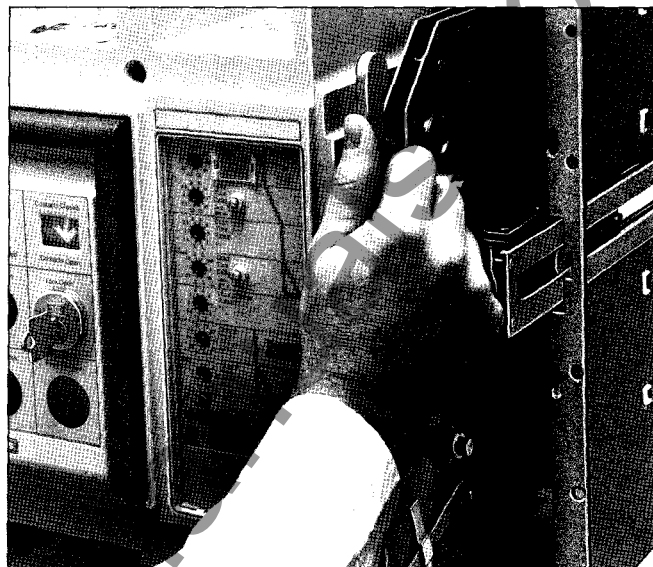
3.) Pump the racking pump handle until the moveable drawout element has reached the test position.
