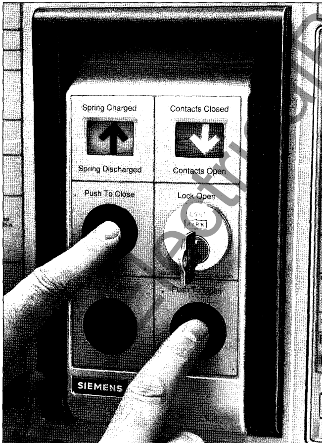
Discharging energy in the stored energy mechanism.
