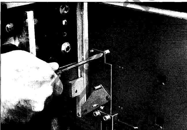
5.) Install top shutter section with #6-32 x 1/4" screws and lock washers, to the sides of the stationary drawout element.
