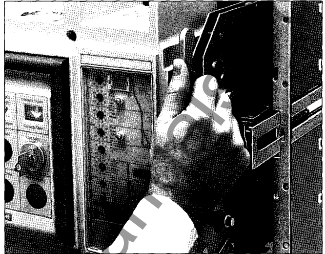
3.) Pump the racking pump handle until the moveable drawout element is in the connected position.
