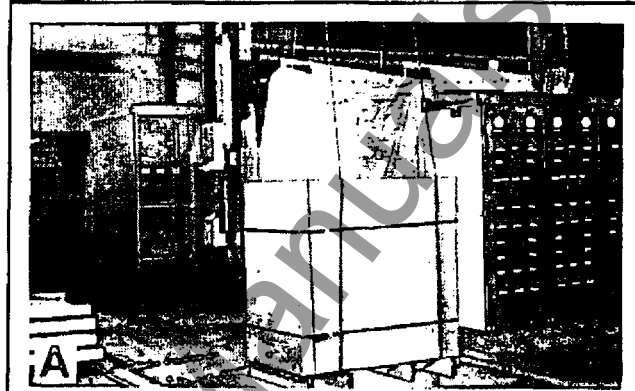
A Move breaker to location with crane or fork lift. Carefully remove carton and protective plastic cover.
