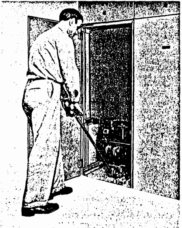
Fig. 19—Pulling Out Circuit Breaker from Housing
