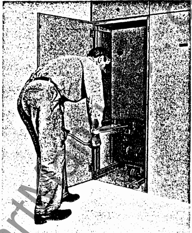
Fig. 17—Racking in Circuit Breaker to Fully Connected Position
