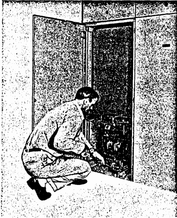
Fig. 16—Levering in Circuit Breaker to "Racked-Out" Position
