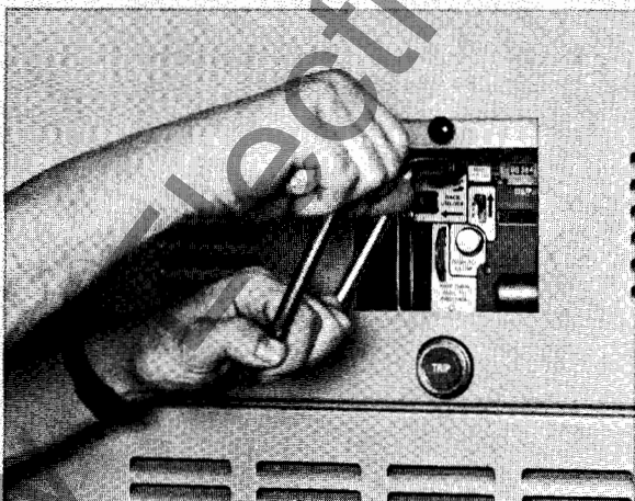
3. Through access port, breaker can be racked into Connected, Test, Disconnected or Out (withdrawn), position.
