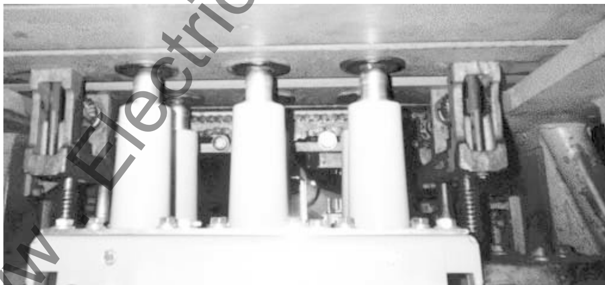
Figure 8. Primary Contact Insertion
