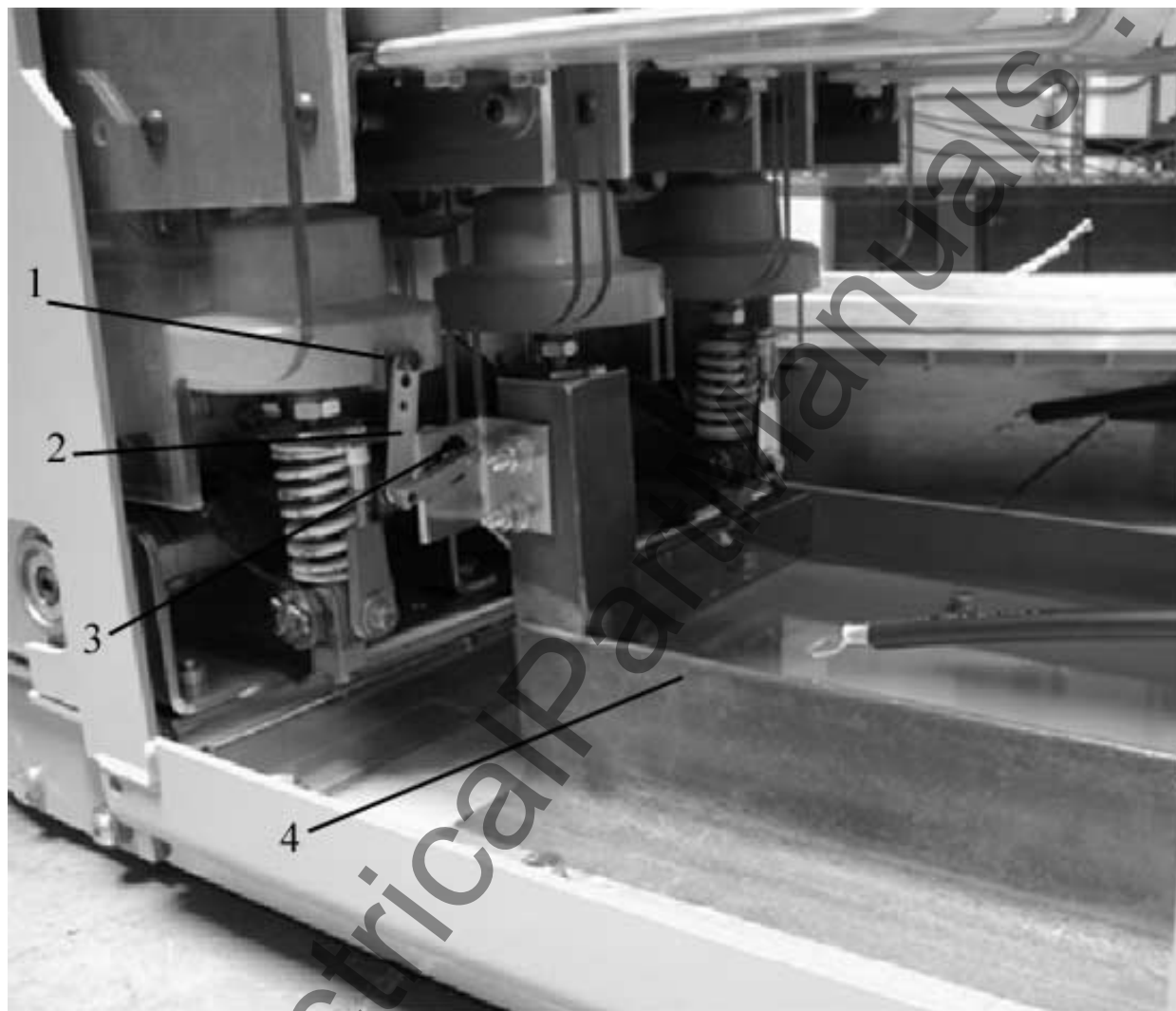
Figure 28. Travel Transducer Installation (Part # 0144D1238G001)
