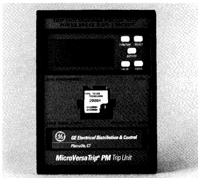
Figure 2. Front view of MicroVersaTrip PM Trip Unit (series RMS9D).
