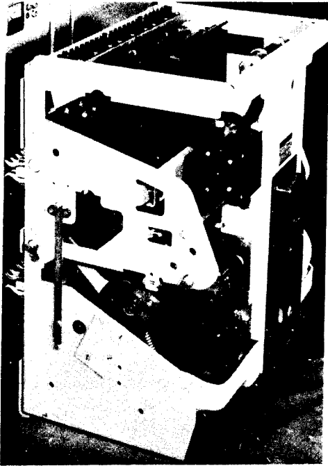
Fig. 17A (8035634) Place Breaker In Front Of Proper Compartment. Operate Drawout Mechanism To Disconnect Position.
