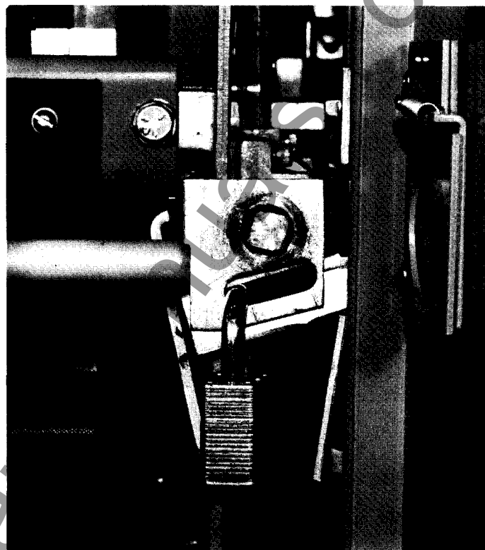
Fig. 7-7. Racking mechanism padlock device (AKR-75/100 breakers)
