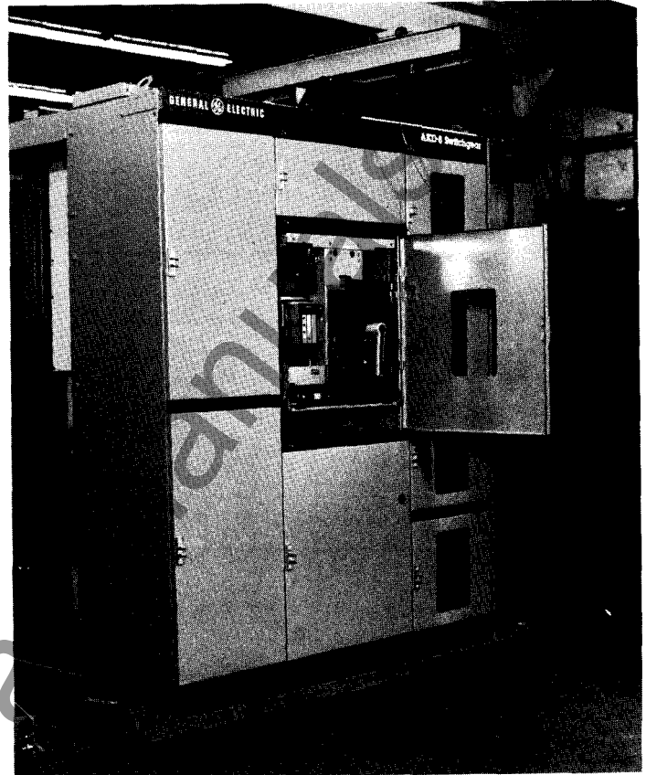
Fig. 5-9. Push the breaker in completely. Close the door.
