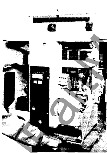
Fig. 33 Drawout Tray In Position To Receive AK-50 Breaker
