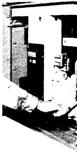
Fig. 38 Racking Handle At End of Fifth Stroke
