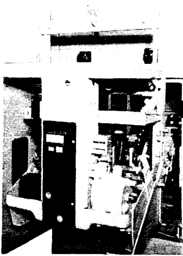
Fig. 32 AK-50 Breaker Raised To Compartment Level
