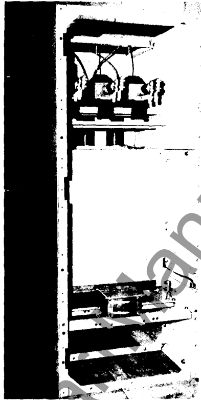
FIG. 27 (8918527-A) REAR VIEW OF UNIT SHOWING GROUND SENSOR TRANSFORMERS
