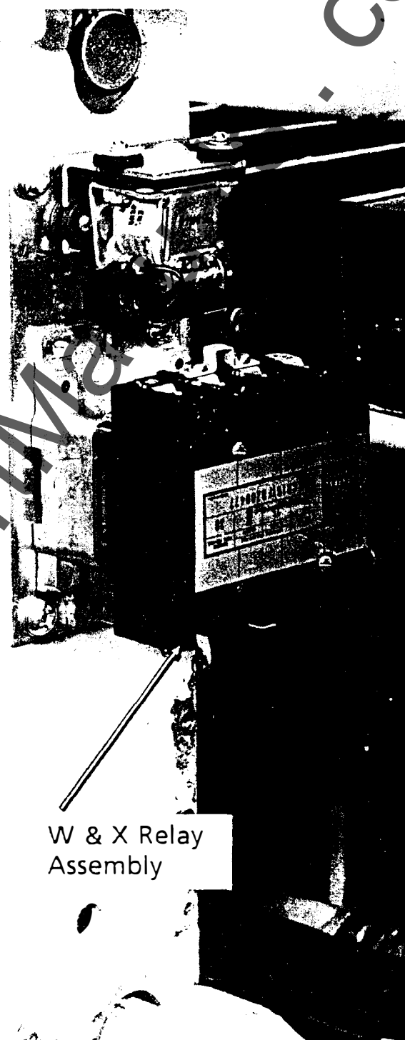
Fig. 14 — W & X relay assembly installed on standard close breaker.
