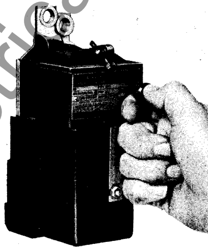
Fig. 127. Checking travel distance of series overcurrent tripping device
