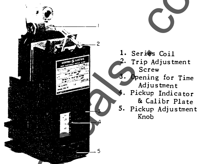
Fig. 16 EC-2 Overcurrent Trip
