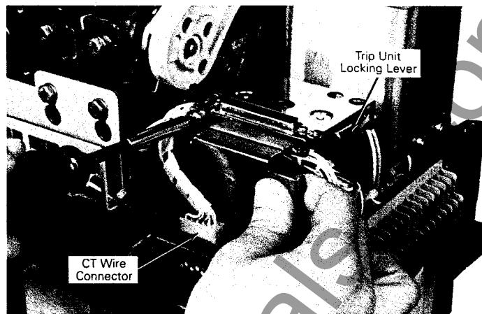
Figure 4. Removing the screws on the trip unit riser bracket.
