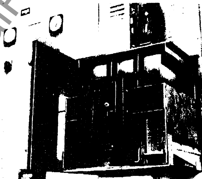
Breaker assembly withdrawn from cell.
