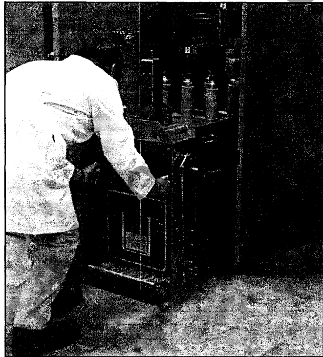
Figure 4-5 Insertion of AM-VR (AM-4.16-VR-250-1200A shown)
