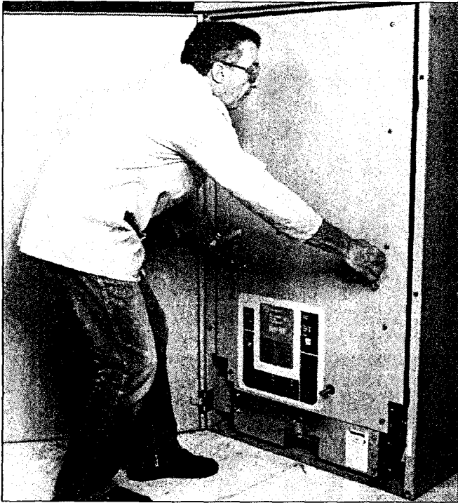
Figure 4-10 Positioning of 7.5 or 15 kV DHP-VR Breaker
