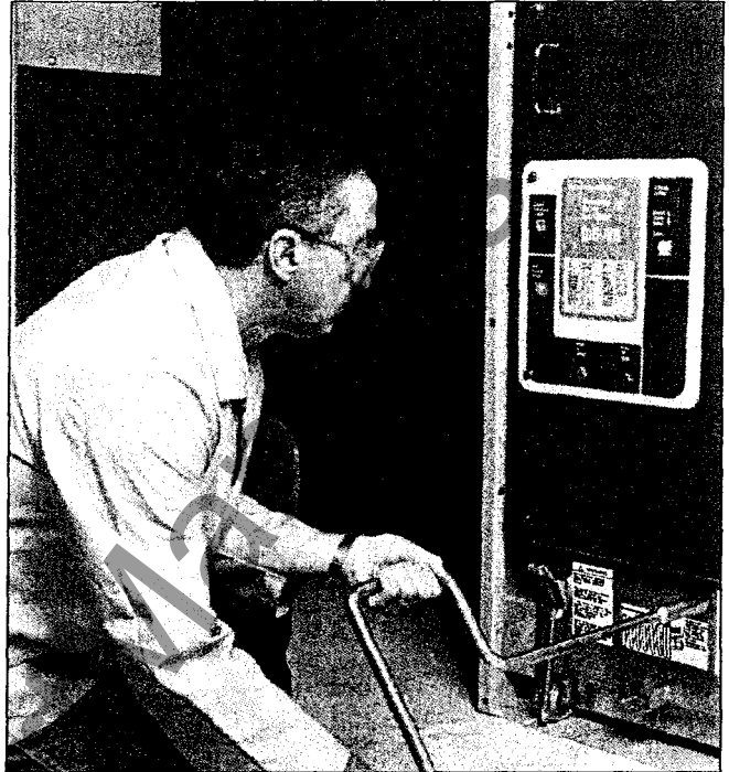
Figure 4-13 Levering 5 kV Breaker to Connected Position
