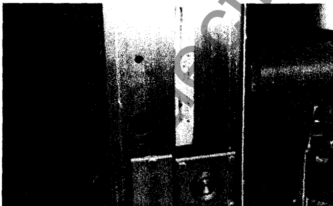
Figure 6-18 Place Tape on Right Side Panel of Breaker
