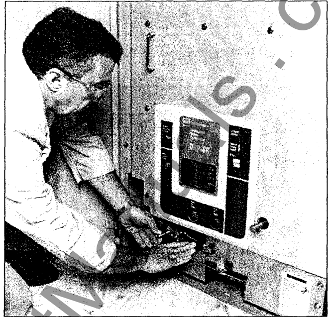
Figure 4-12 Final Engagement of 7.5 or 15 kV Secondary Contact
