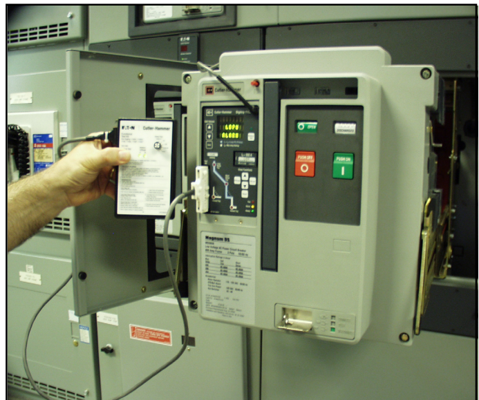
Figure 1.3 Testing Digitrip 1150 with Magnum Breaker in Disconnected Cell position
