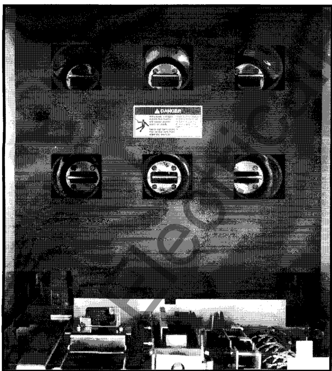
FIG. 8 CT BARRIER (SHUTTERS BLOCKED OPEN)
