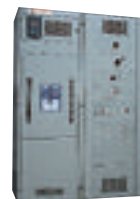
Low Voltage Switchboard
