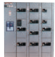
Motor Control Center
