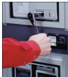
The breaker can be conveniently racked in or out, stopping at the various positions with the door closed.
