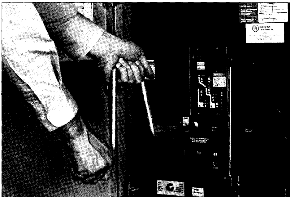
DSII Breaker Levering Operation
