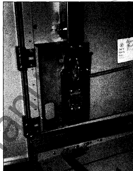
Key Interlock and Linkage
