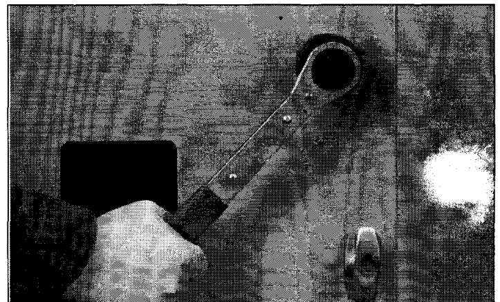
Figure 15. Arcflash Reduction Maintenance Switch Mode Selector Switch Hole Being Cut in the Mounting Surface.
