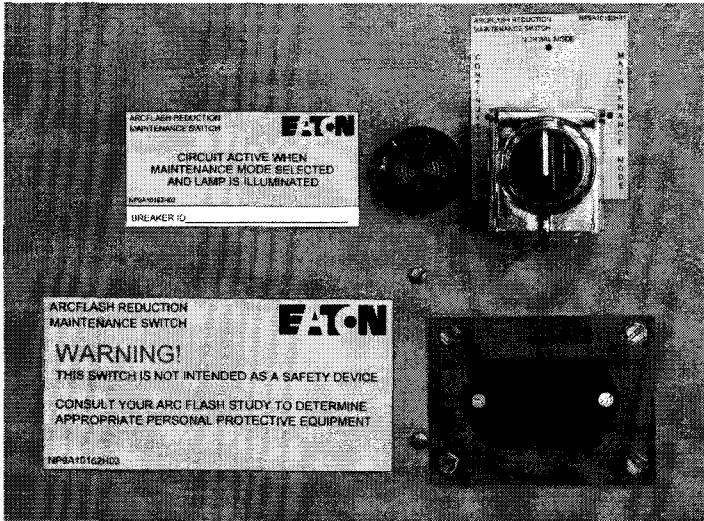
Figure 24. Warning and Circuit Active Labels installed on the Mounting Surface.
