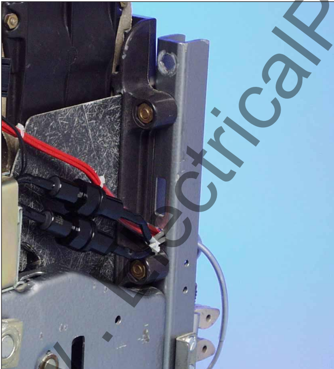
Fig. 48 Correct Positioning of the HV Fuses
