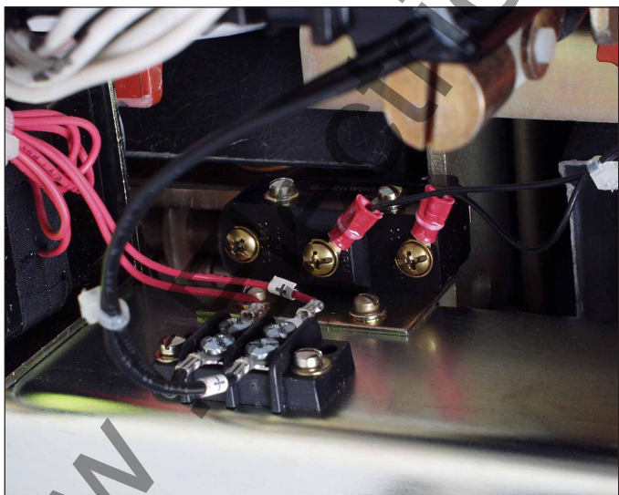
Fig. 65 Connecting the Auxiliary Switch
