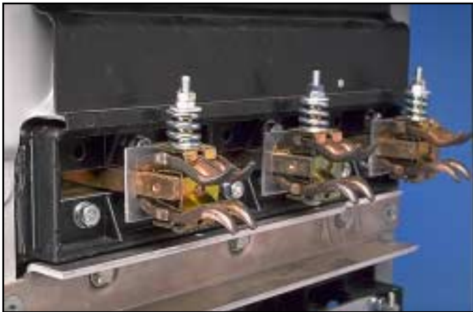
Fig. 13 Breaker Stabs Drilled and Tapped for HV Wire Connection.
