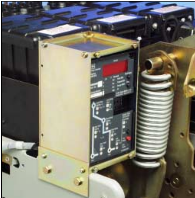
Fig. 39 Overview: Trip Unit Installed on the Breaker.
