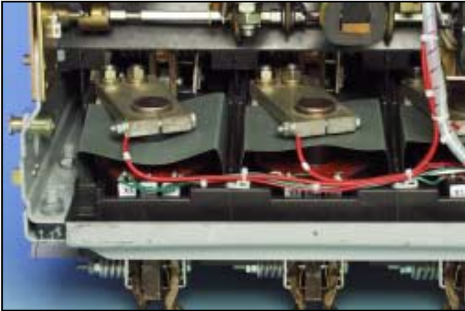
Fig. 23 PT Wires Attached to the Copper Connectors.
