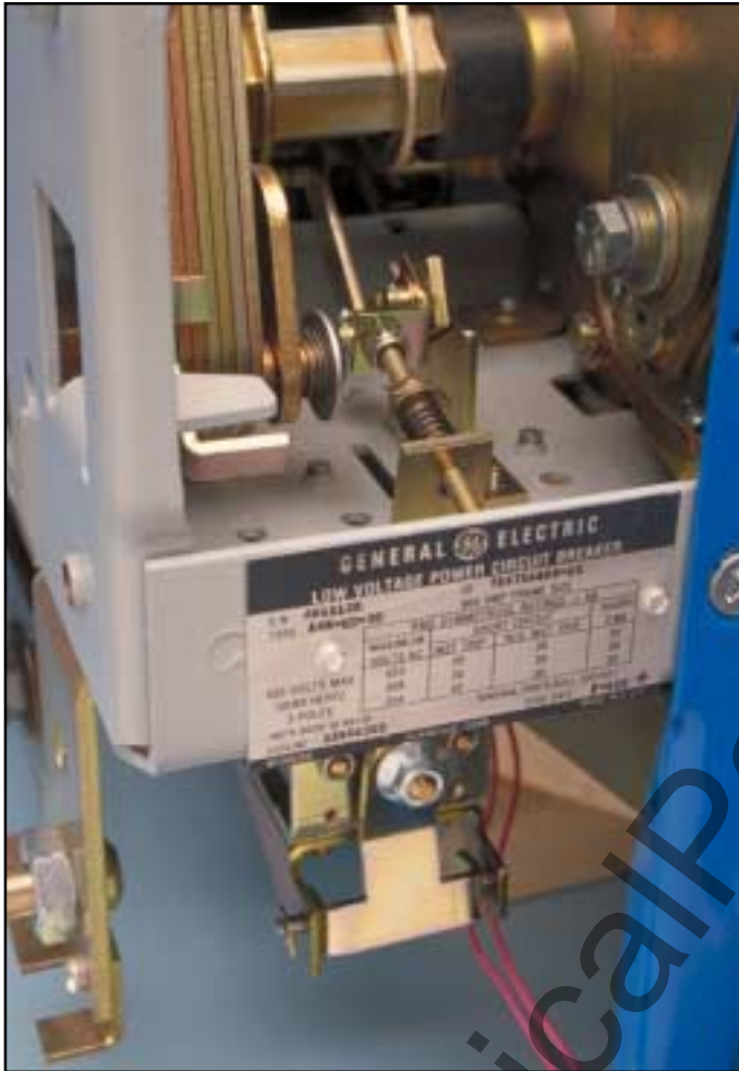
Fig. 28 DTA and Reset Assemblies Installed in the Breaker.
