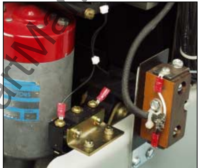
Fig. 46 Auxiliary Switch Wires Connected to the Auxiliary Switch.
