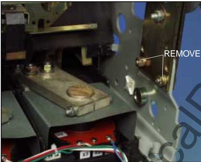
Fig. 11 Hardware to be Removed from the Right Side of the Breaker.
