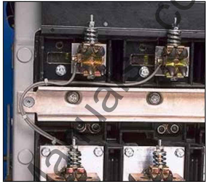
Fig. 14 Routing of the HV Line Side Wires.
