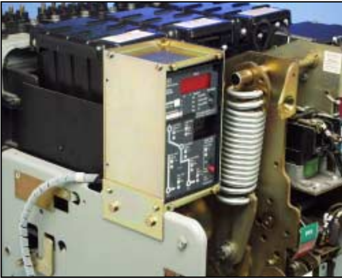
Fig. 47 Trip Unit Assembly Mounted to the Left Breaker Frame.
