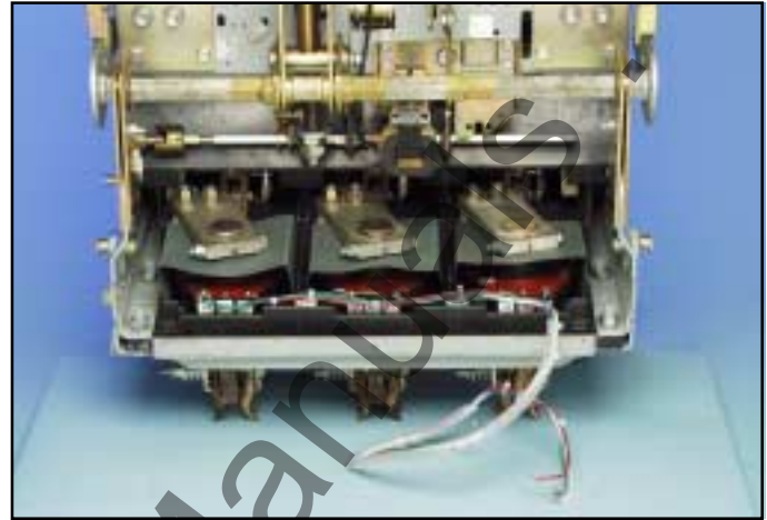
Fig. 2 Overview: Sensors and Sensor Harness Installed in the Breaker.
