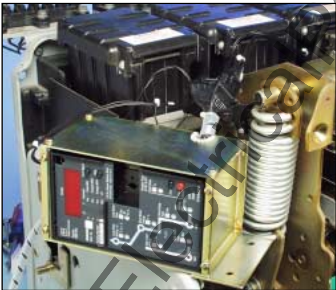
Fig. 45 Harnesses Connected to the Trip Unit and External Harness.
