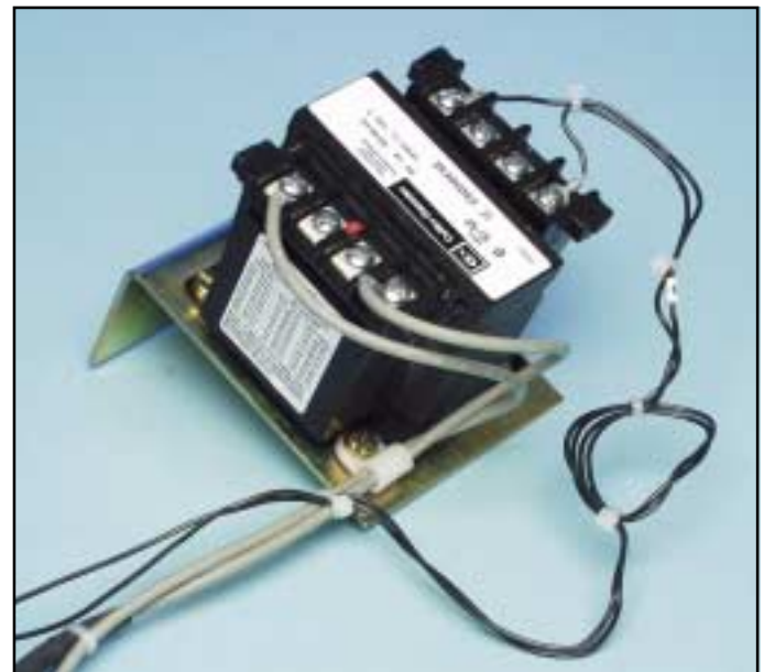
Fig. 10 HV and CPT Wires Connected to the CPT.
