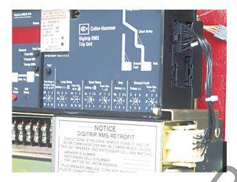
Step 5: Installing the Trip Unit
